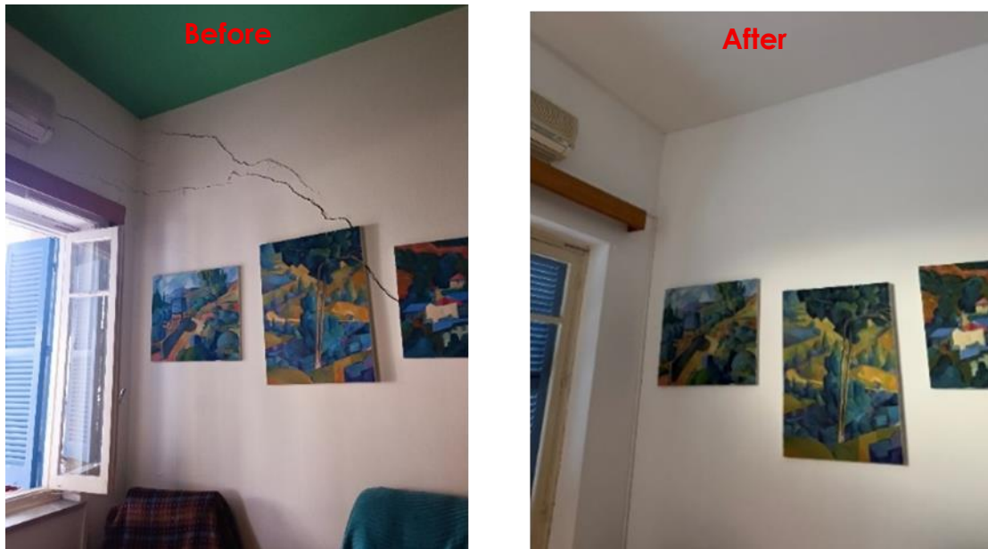
Figure 4: Crack Repair in Load-Bearing Masonry building
