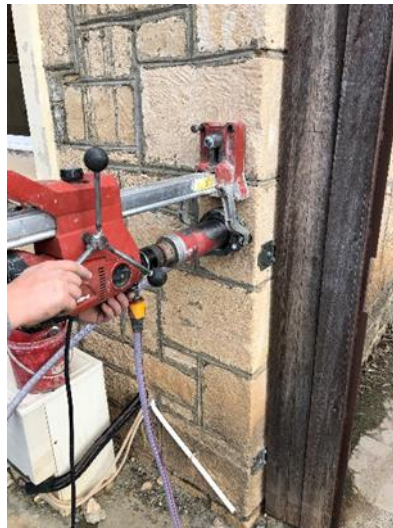
Figure 3: Core extraction
