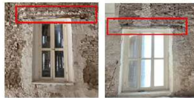
Photo – 1: Existing timber lintels found above openings
