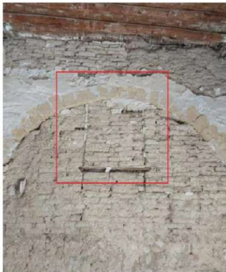
Photo – 2: Founding of larger window that will be strengthened with two (2) timber ties.
