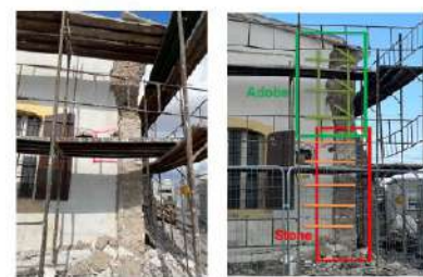
Photo – 8: Existing S.E. corner wall typology - bottom half part made of stone masonry, upper half part made of adobe masonry
