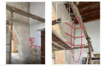
Photo – 4: Stitching of cracks found at the corner connection of the masonry walls by means of 3 pairs of timber corner elements (W6.0)
