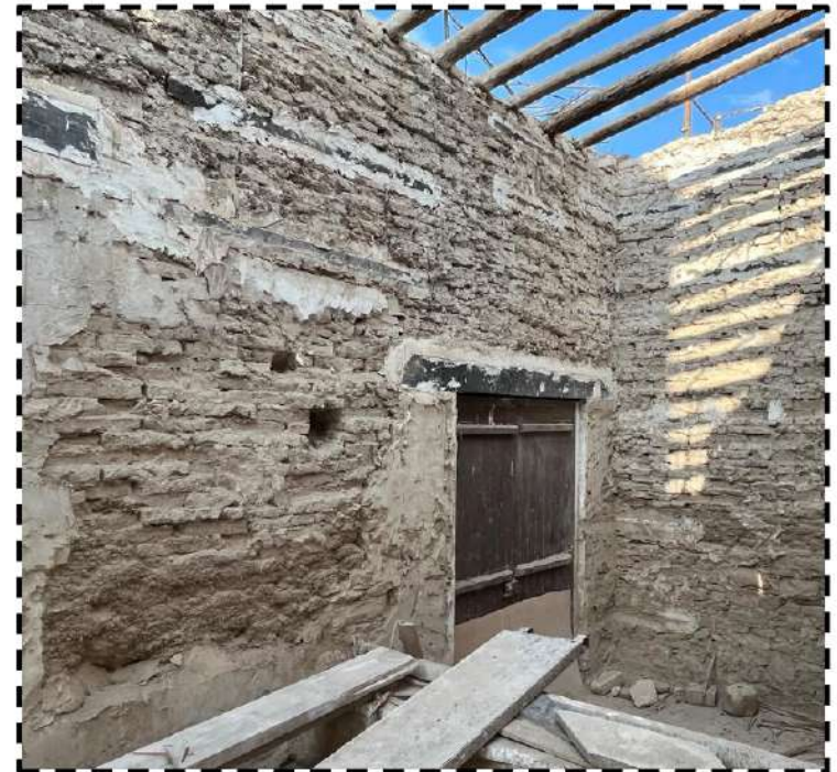
Photo – 3: Founding of small window that will be strengthened with one (1) timber tie.
