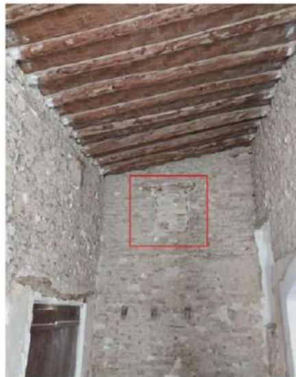
Photo – 3: Founding of small window that will be strengthened with one (1) timber tie.
