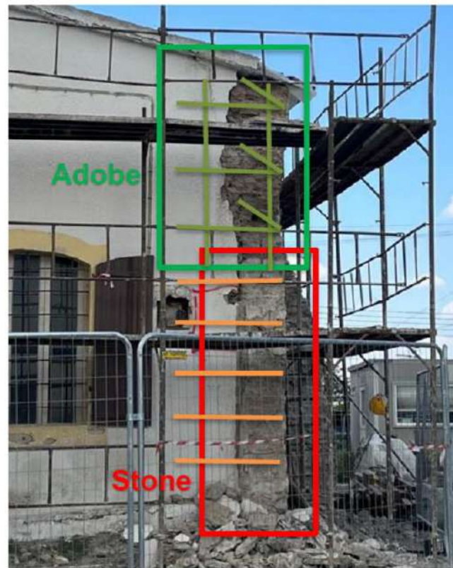
Photo – 8: Existing S-E corner wall typology – bottom half part made of stone masonry, upper half part made of adobe masonry
