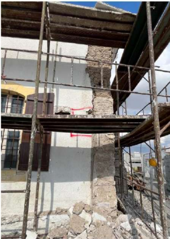
Photo – 8: Existing S-E corner wall typology – bottom half part made of stone masonry, upper half part made of adobe masonry
