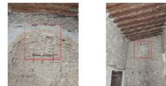
Photo – 2: Foundation of larger window that will be strengthened with two (2) timber ties.
